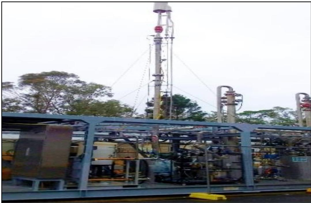
Figure 7: 1350 Kg/d hydrogen production module. Source: Synergen Met Pty Ltd website
