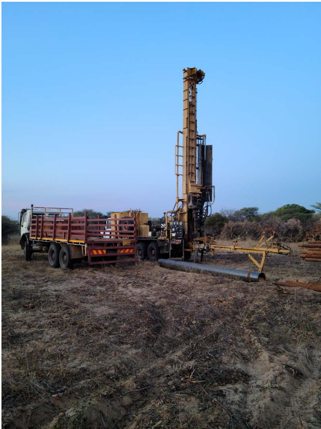
Rig on location
