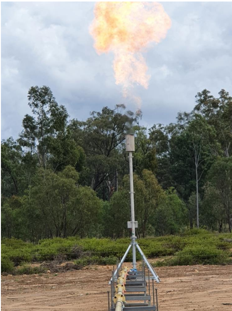
Gas flare at Venus 1 Pilot well during pressure drawdown
